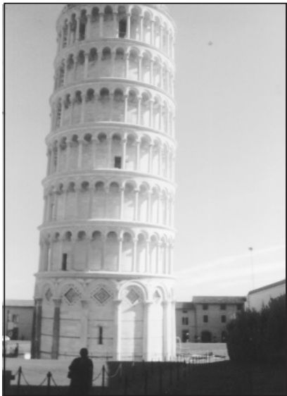
Leaning Tower of Pisa
